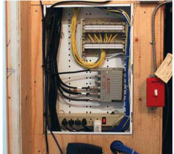
The technician spent four hours redoing the cable TV and six more for the LAN and TEL services, Ohman estimates. The modem, computer switch and router remain below the enclosure, which “was half as big as it should have been,” notes Ohman.
